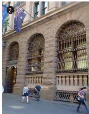
2. Inactive facade of heritage building. Paspaley
